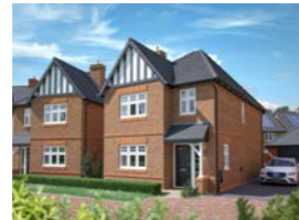
The Rosewood 4 bedroom homes
